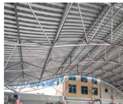
The 4" deep ribs provide excellent strength and spanning capability.
