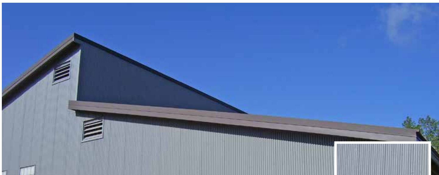
Allegan Water Treatment Facility, Allegan, MI, USA
