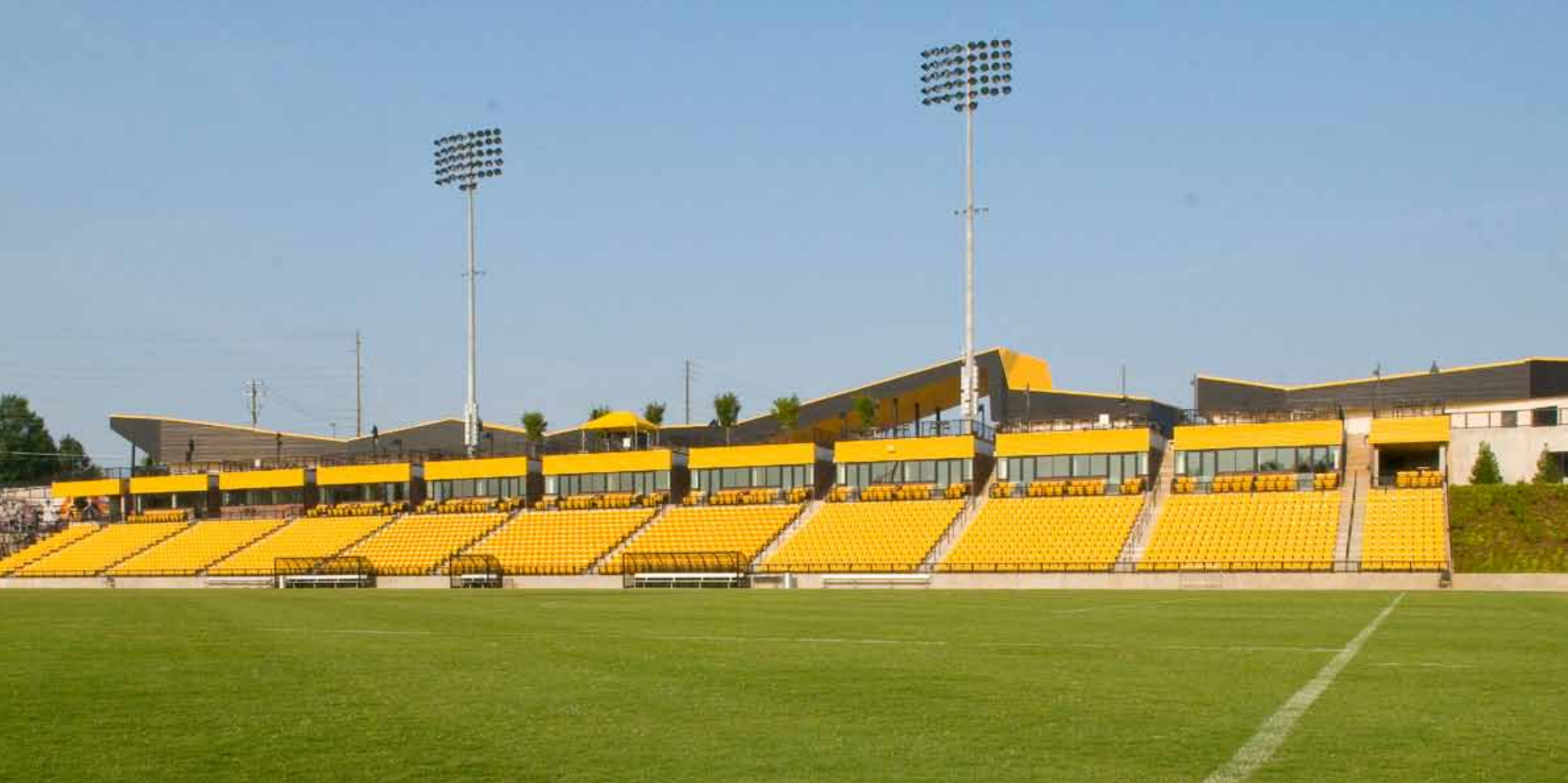
Kennesaw State University Women's Soccer Stadium Kennesaw GA, USA
