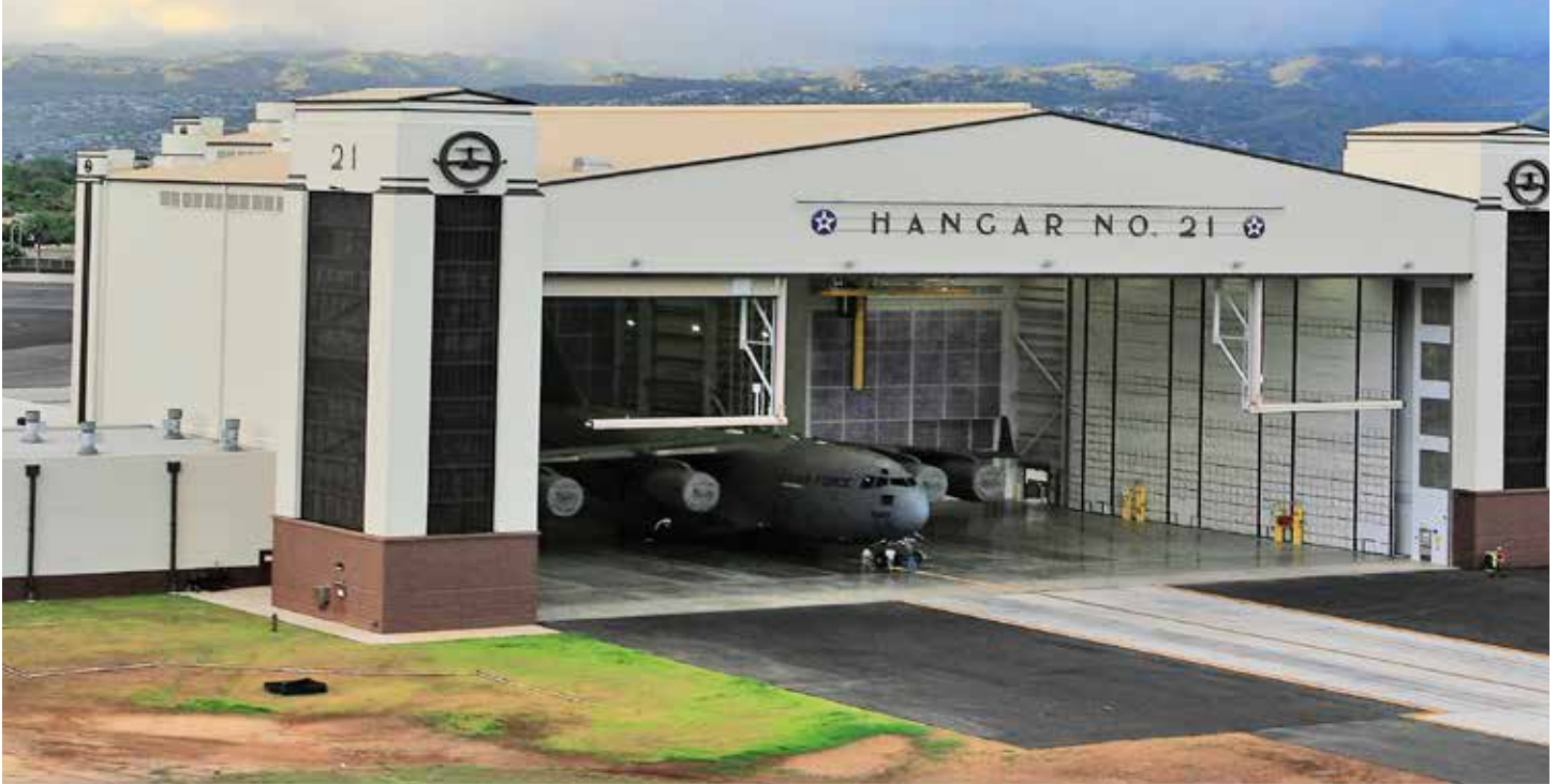
Hickam Air Force Base, Oahu HI, USA featuring Mighti-Rib® and V-Beam
