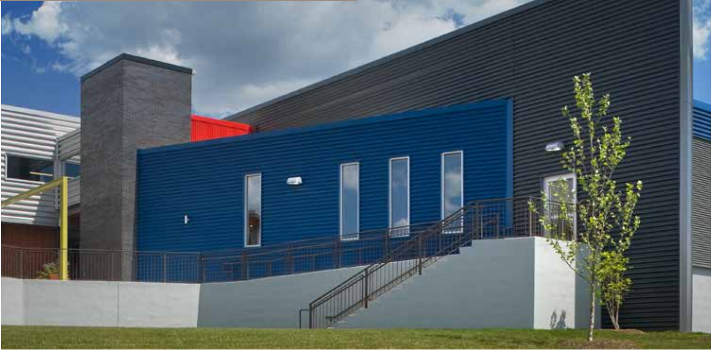
Coleman Park Community Center, Nashville TN, USA featuring Deep Rib II and V-Beam
