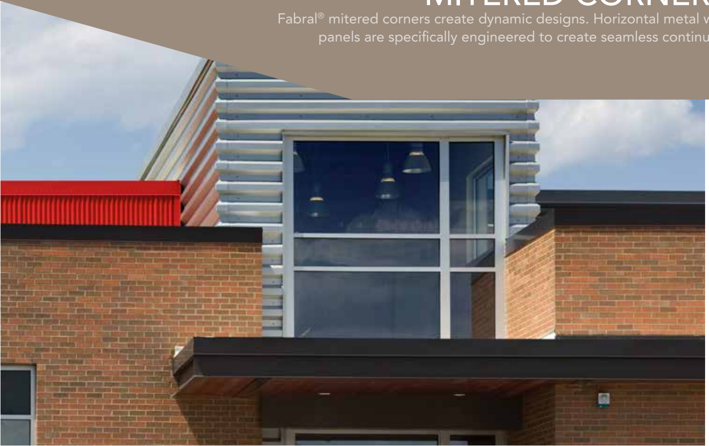
Coleman Park Community Center, Nashville TN, USA featuring Deep Rib II and V-Beam
