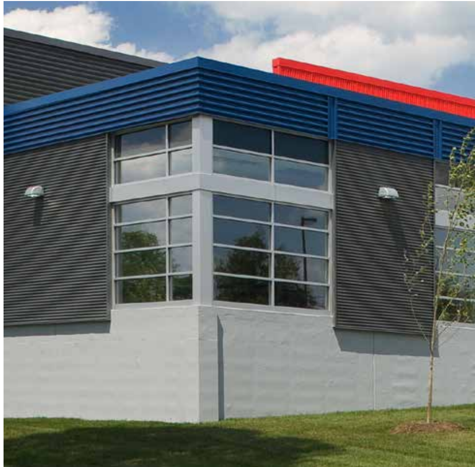
Coleman Park Community Center, Nashville TN, USA featuring Deep Rib II and V-Beam
