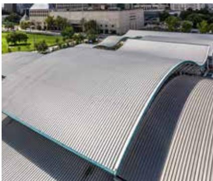
Although not shown in this particular project, Deep Rib IV can be field formed to accommodate lengths longer than Fabral's maximum 45'.
