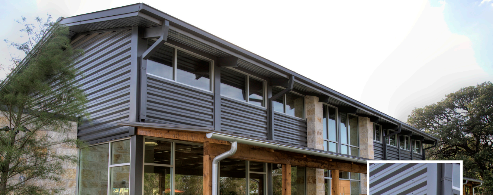
4.0 Wine Cellar, Fredericksburg, TX, USA
