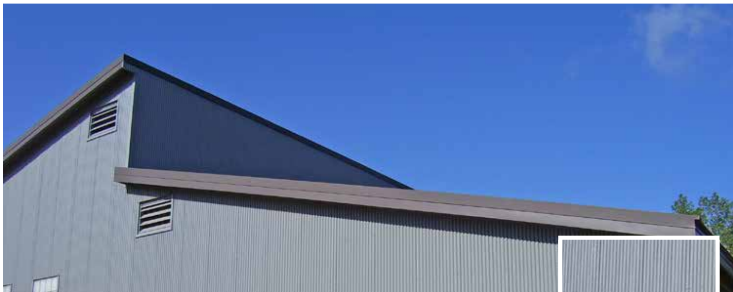
Allegan Water Treatment Facility, Allegan, MI, USA
